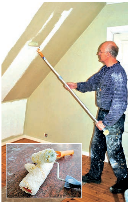
It is best to use a yarn roller to paint wallpapered walls. Note: The roller should roll easily over the surface.
