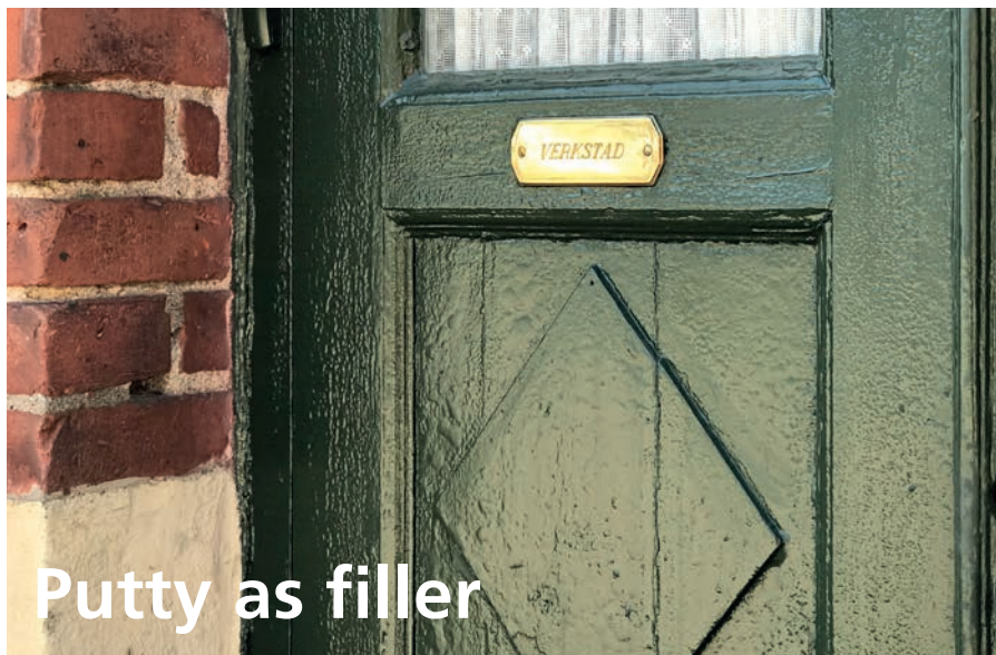
Door from 1926. Easy "anti-aging" measure for 100 years. Linseed Oil Putty in cracks. Painting an old surface with new Linseed Oil Paint.
