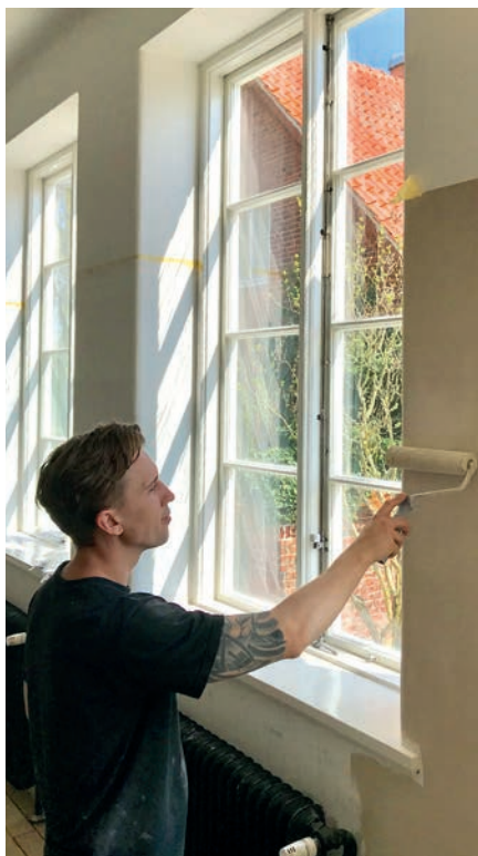
Fill and paint with Linus Wall Paint. Use a yarn roller or brush. Spread filler on whole surface or roll with Linus + ground pumice.
