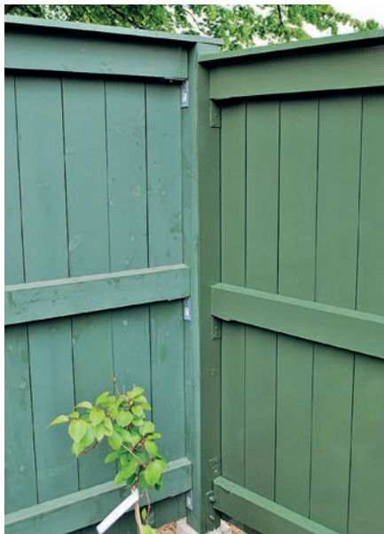
First and second coat. FINISH PAINTING! At least two and preferably three fully covering coats.
