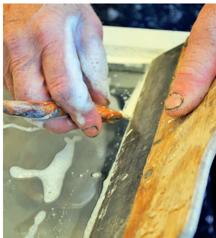
Cut the edges of the putty rebates in a weak soap and water solution.
