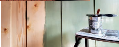
Treat knots in wood with shellac. Paint outdoors and indoors, 2–3 coats.
