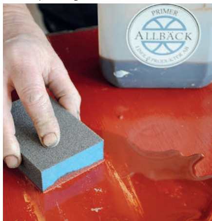
Wet-sanding with Primer will remove a raisin-like texture.
