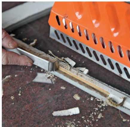
Putty Lamp to remove putty. It can also be used to remove paint to some extent.
