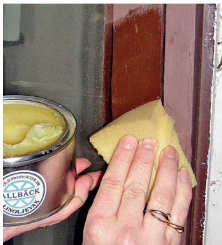
Linseed Oil Wax on matte painted surfaces or untreated wood.
